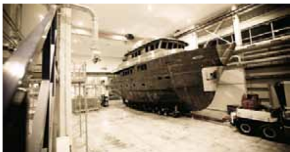
▲ A Darwin 86 under construction
